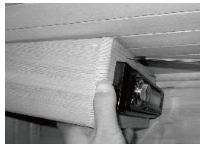
FIG-17 Screwing in the Radio Wood Housing
