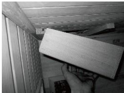
FIG-16 Installing the Radio Wood Housing
