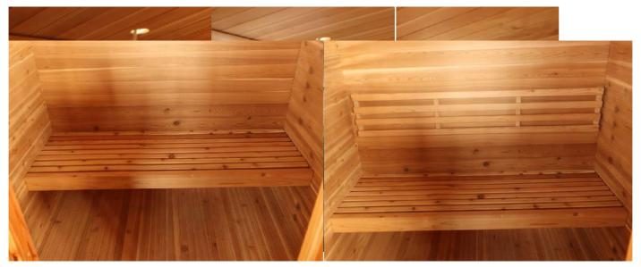
9. Place the seat bench onto the wall supports and attached the back rest using the included screws.
