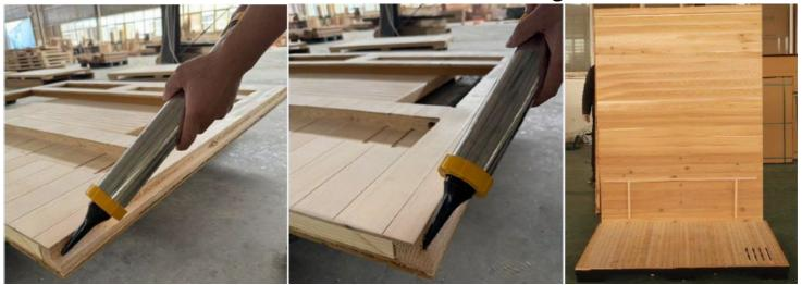
3. Attach right and left walls using the pre-installed buckles
